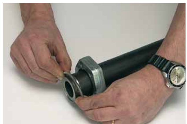
Install the retain ring onto the pipe.
